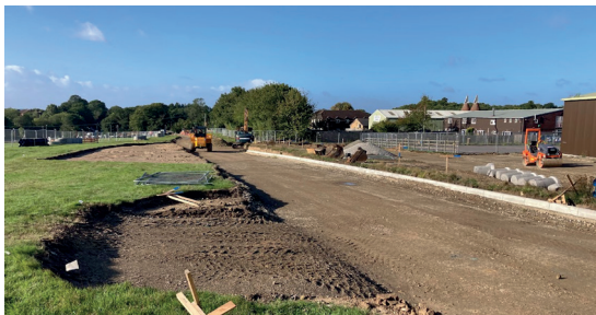
The New Access Road is well underway
