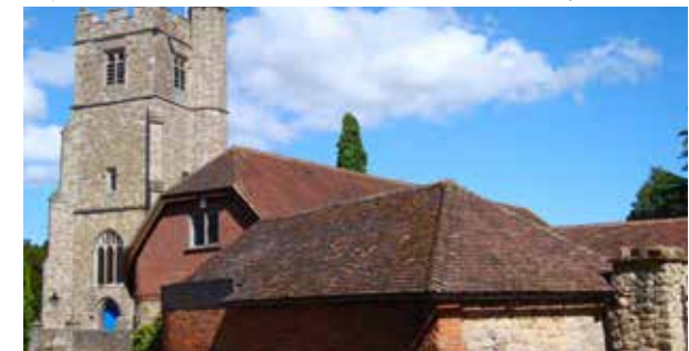
Figure 12: Holy Cross Church with Mote Hall Barn in the foreground
