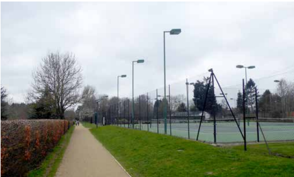
Figure 30 The tennis courts are higher than the adjacent bridge path
