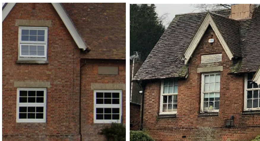
Figure 4 - example of UPVc window and traditional window
